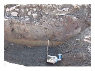
Photo 6 - View at trenchwall materials NE of cofferdams; note: top of gravelly fill below surface soil contact with dredged fill.
