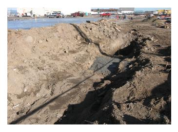
Photo 5 - View looking NE along new sanitary sewerline trench; cofferdam in central portion of photo.
