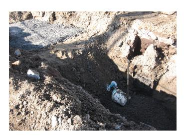
Photo 4 - Controlled-density fill (CDF cement) cofferdam installed over and around new sewerline and gravelly fill.
