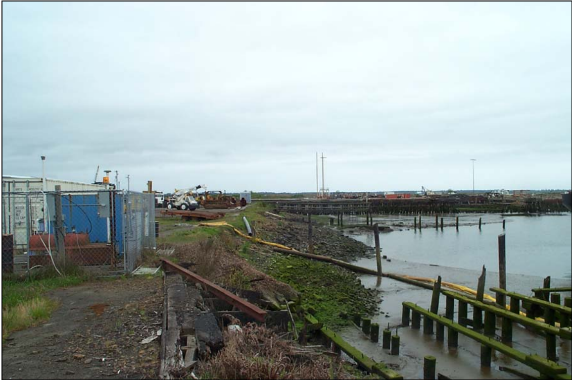
Photograph 23 - Looking southwest along margin of Slip 2. Note riprapped banks.
