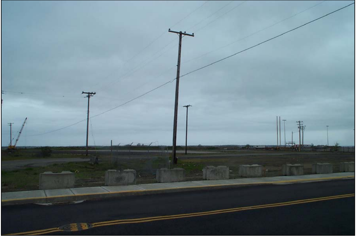
Photograph 15 - Looking west at former McCall Oil (Chevron) Bulk Plant location.
