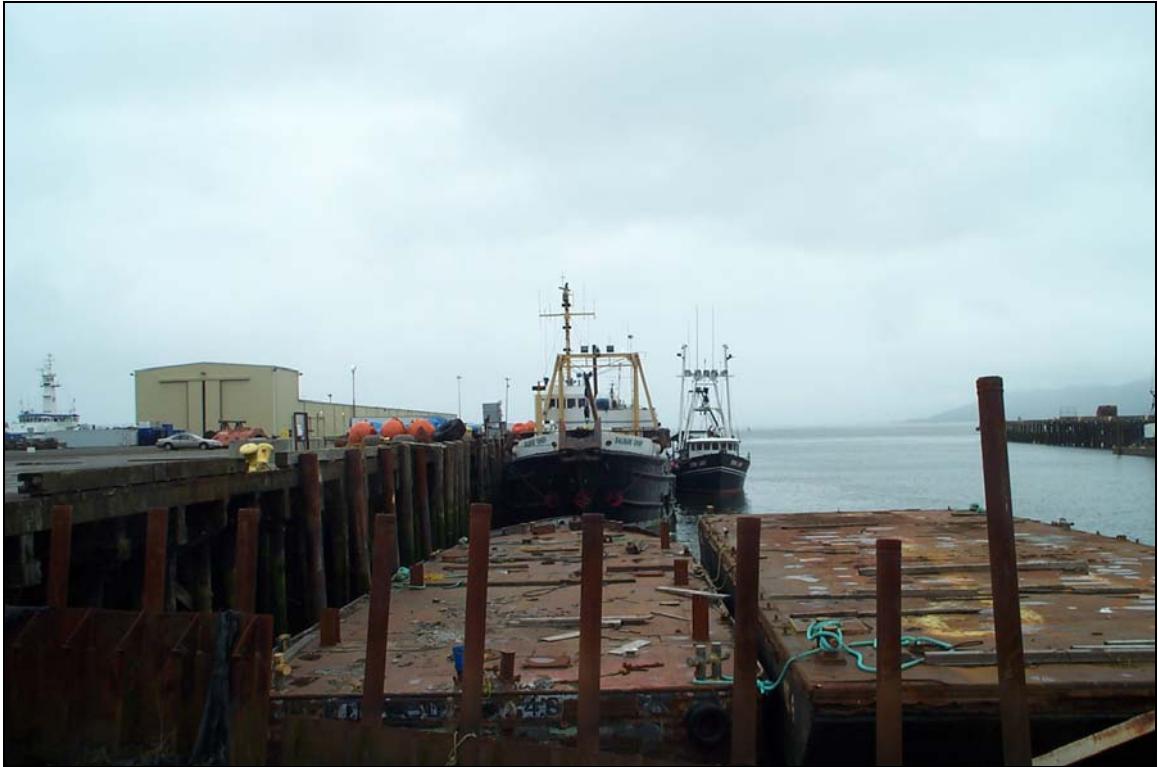
Photograph 31 - Looking northwest along west side of Slip 1. Note wooden docks, pilings, barges, and ships docked in slip.
