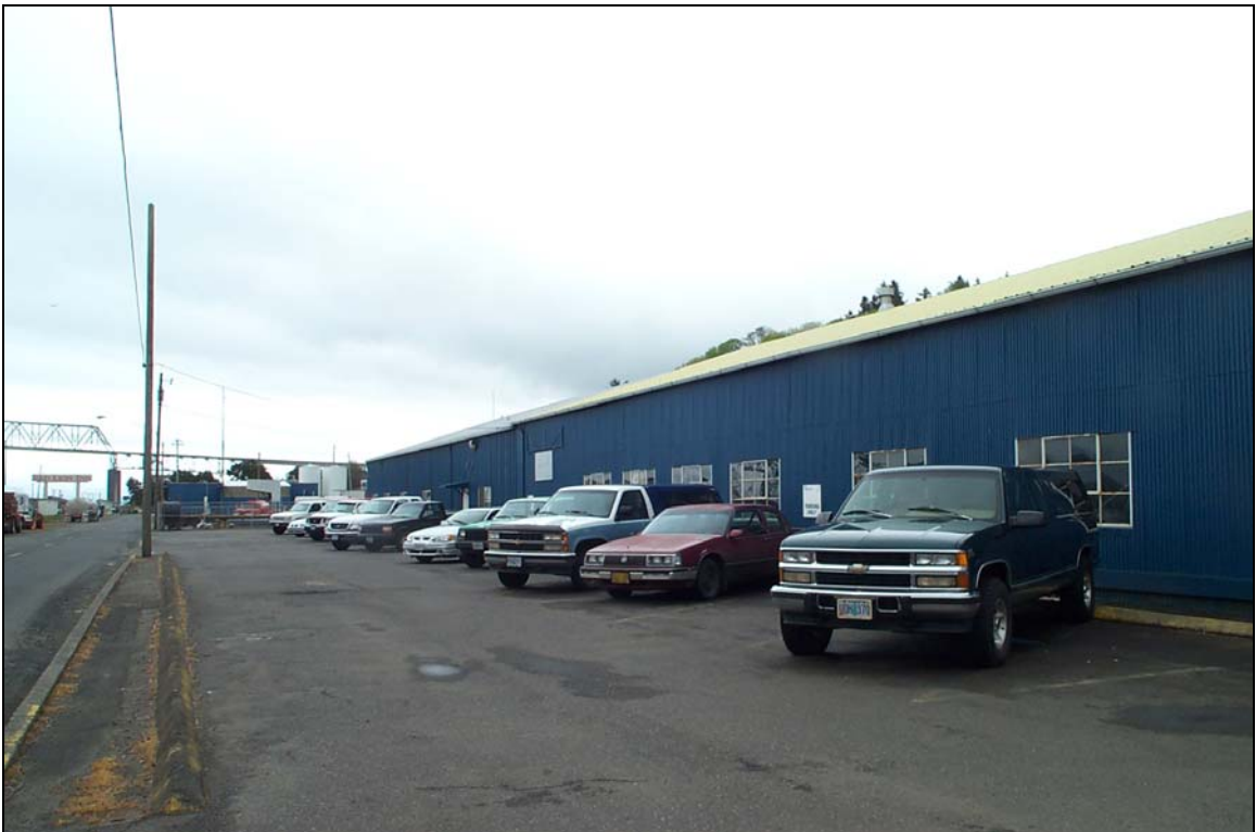
Photograph 10 - Looking northeast towards Qwest facility on Industry Street.
