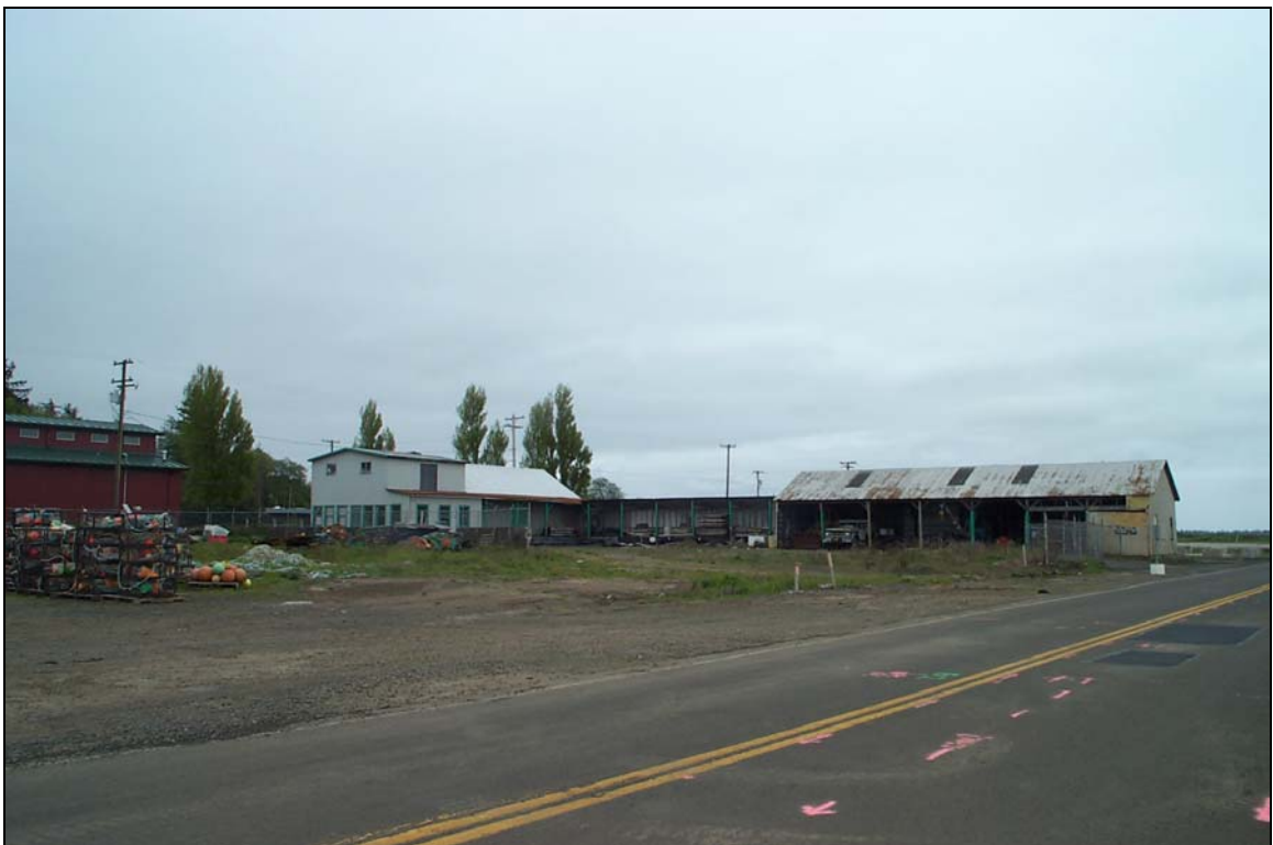
Photograph 18 - Looking south at former Niemi Oil Bulk Plant location.
