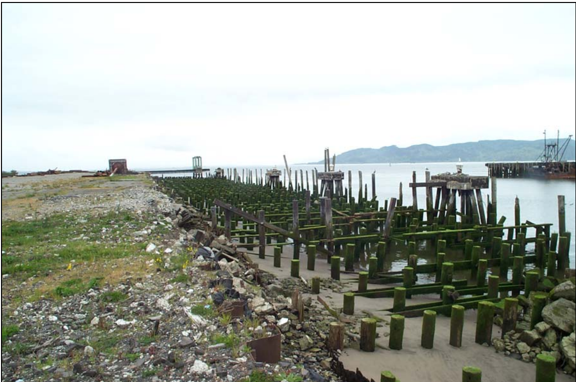
Photograph 28 - Looking northwest at disturbed habitat in Slip 2 and on Pier 3.
