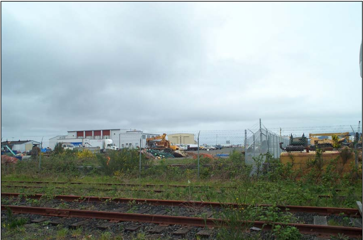
Photograph 8 - Looking northwest toward former steelworks property.
