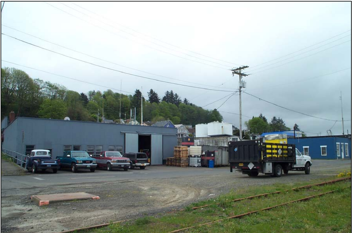
Photograph 6 - Looking south at Delphia property on Industry Street.
