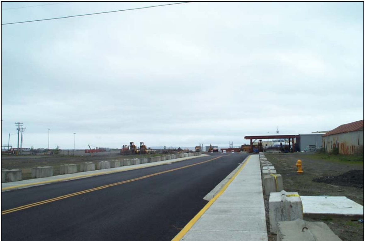
Photograph 16 - Looking northwest along Hamburg Avenue toward Slip 2.
