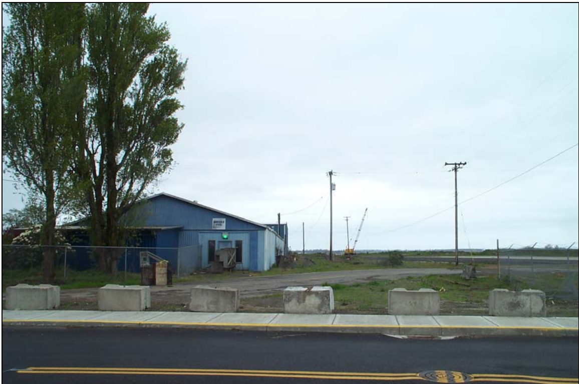
Photograph 14 - Looking southwest along boundary of former McCall Oil (Chevron) Bulk Plant location.
