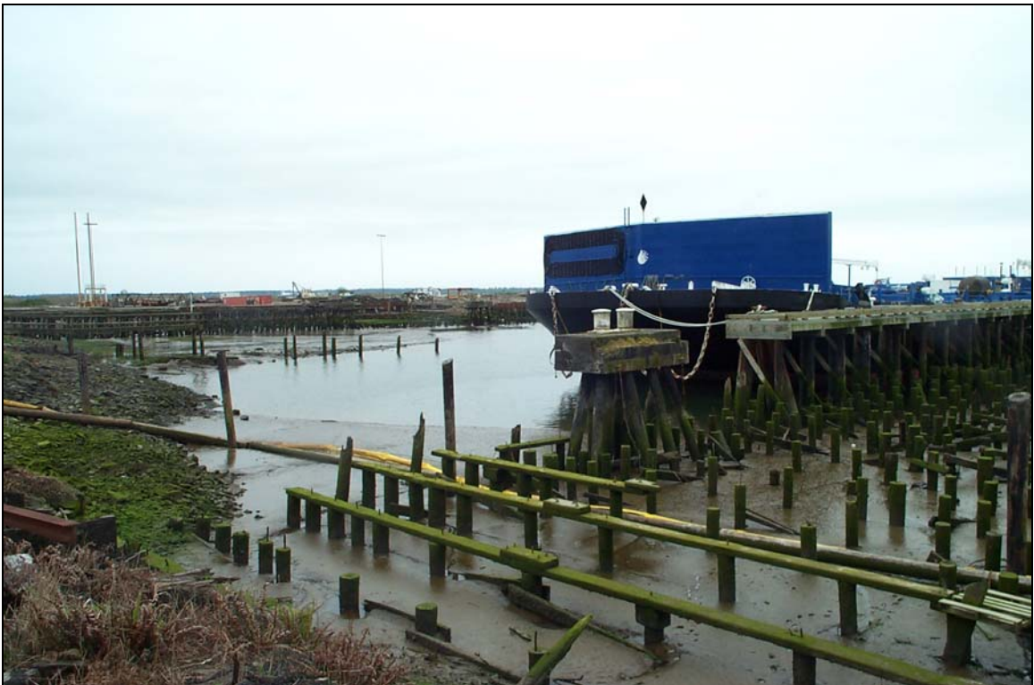
Photograph 22 - Looking west along margin of Slip 2. Note Oregon Responder Barge moored on northeast side of slip.
