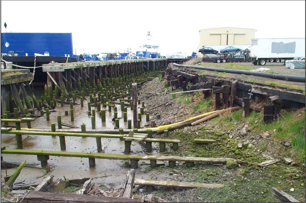
Photograph 21 - Looking northwest along Slip 2 and seep area. Note containment boom and charred area of historic dock fire.
