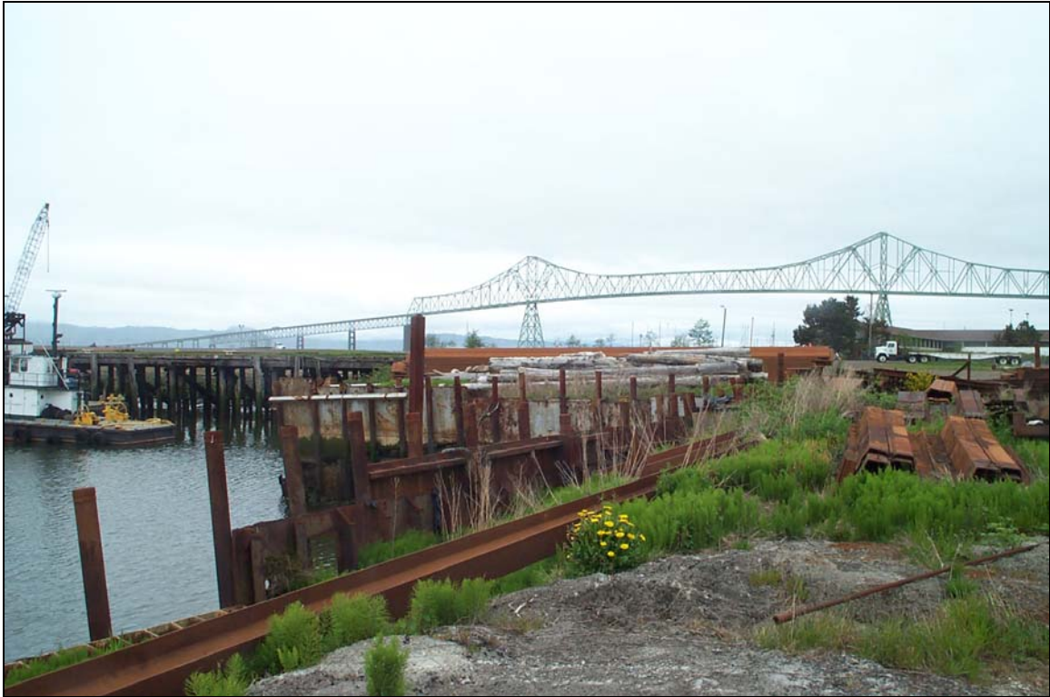
Photograph 33 - Looking northeast along face of Slip 1. Note weedy vegetation and sheetpile bulkheads.
